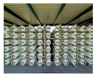
Reverse Osmosis Membranes at West Basin Municipal Water District, Brewer Desalination Facility. Desalination of local brackish groundwater helps reduce the Region's dependence on imported water.
